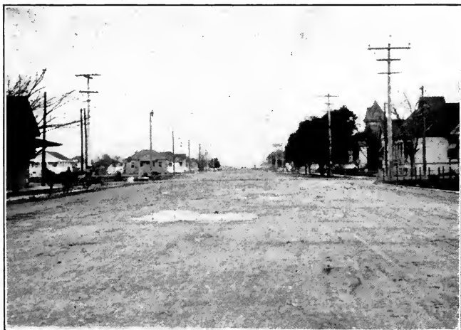
A STREET OF NEEDLESS WIDTH IN A RESIDENCE SECTION Wasteful of valuable space, and expensive to repair and to maintain. Houses crowd close to the street, because lots must be made correspondingly shallow.
